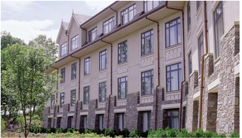
32 Window Surrounds, Soffit
